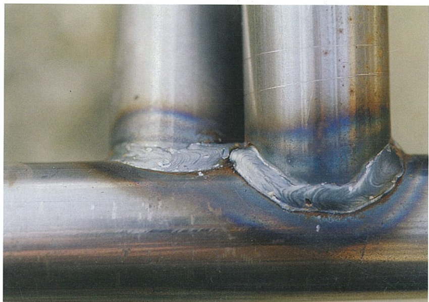
Fig. 4.20. Fully welded frame tube joints. (Steve Williams)
