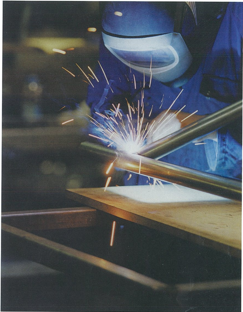
Fig. 4.19. Starting to fully weld the frame. Remember to weld alternate sides to minimise distortion. Spot the deliberate mistake – the welder should be wearing thick gloves! (Steve Williams)
