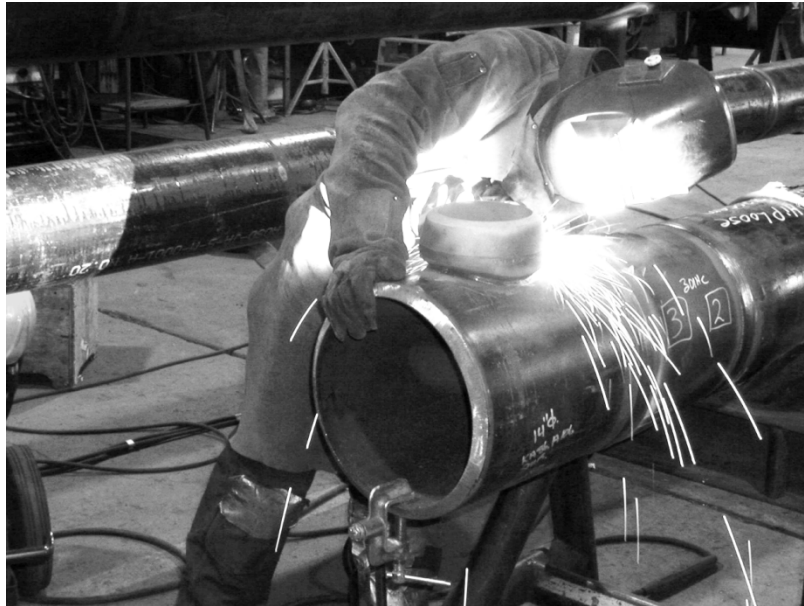
Figure 7 - Protection from sparks and slag.
