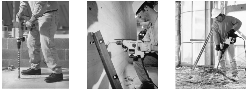
Figure 44 - Hammer drills in use. (Courtesy Dewalt)
